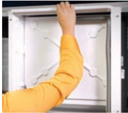
Remove the top plastic cover.
